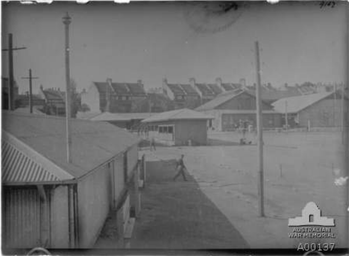
Portion of the Engineers Depot Camp taken from the southeast corner
