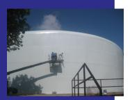
Coatings applied to the water storage tanks provide a protective barrier between the steel and the moisture in the atmosphere.
